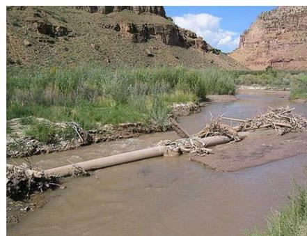
Figure 4: Picture of an exposed pipeline crossing an unnamed western US river.
